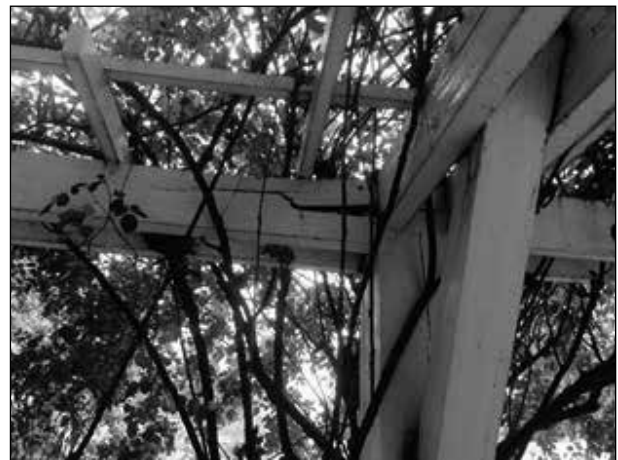
The wooden elements of the Rose Arbor have weathered and deteriorated despite ongoing maintenance.
