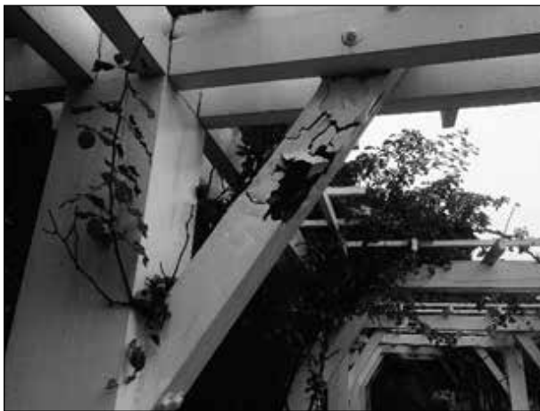
The wooden elements of the Rose Arbor have weathered and deteriorated despite ongoing maintenance.
